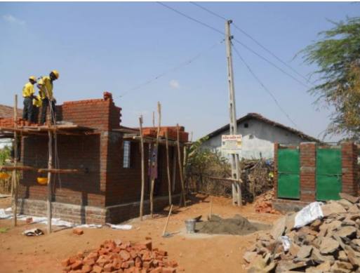
Trainees from ACF's Mason Training Program constructing Galiben's new home.
