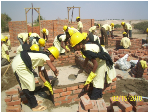
Students of ACF's mason training program build community assets as part of the practical component.
