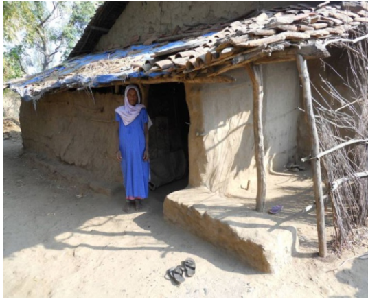
Galiben's home, before ACF's intervention.
